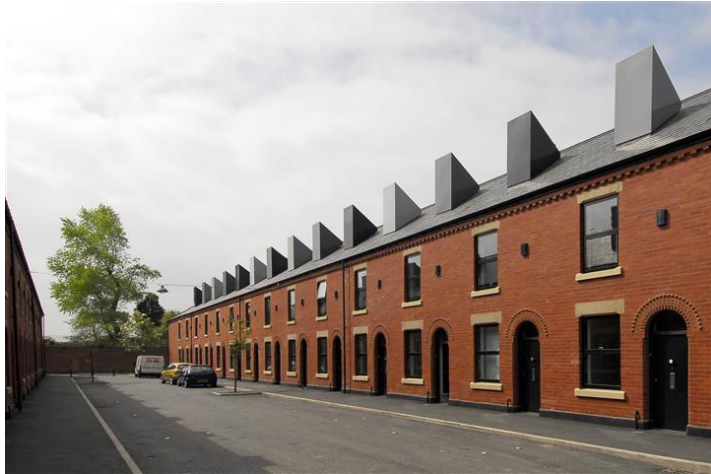
Chimney Pot Park, Salford
